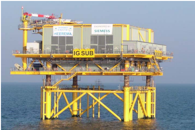
504MW Greater Gabbard in construction
